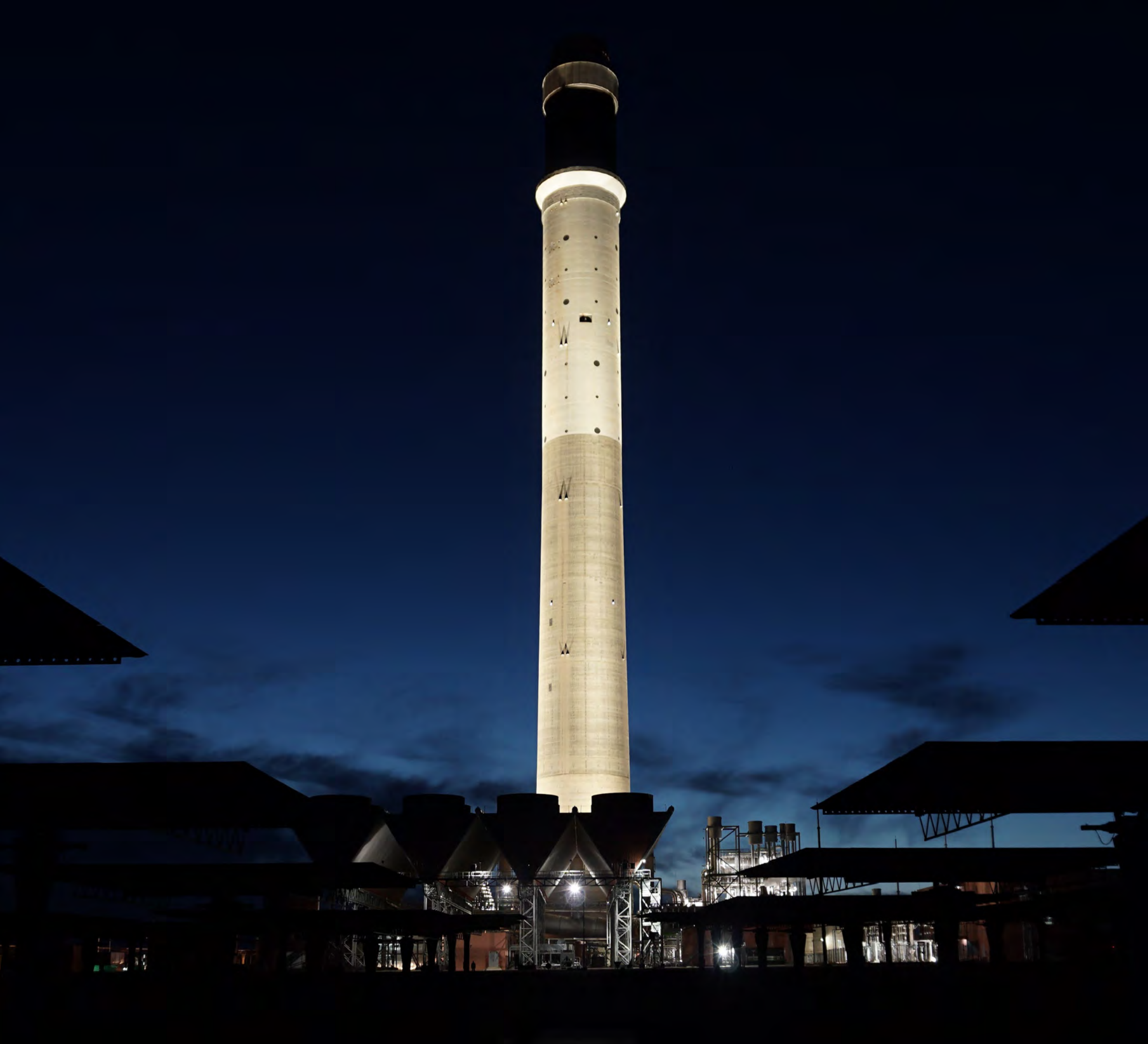
MOROCCO_Noor Tower, Ouarzazate
